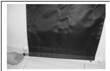
The anchor rail must be fixed securely to the bathroom floor directly opposite the wall-mounted belt housing case.
