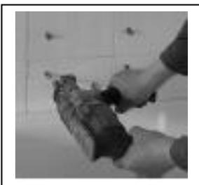
Place the fixing plate against the wall, approximately 11 cm (4.3") raised from the bathtub edge, with one end of the fixing plate near the beginning of the bathtub curve, as it is shown left. Mark six holes through the fixing plate and please make sure that the fixing plate is kept horizontal.
